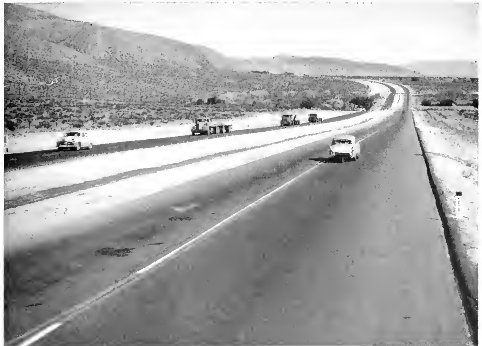
UPPER: Intersection of US 99 and road to Twentynine Palms and Joshua Tree National Monument has been channeled as shown here in the latest contract completed. Snow-capped Mt. San Jacinto, elevation 10,831, in background. LOWER: Note heavy trucks pulling upgrade from Coachella Valley into San Geronio Pass. Before completion of this four-lane section, each truck would have been trailed by five to twenty passenger cars.
